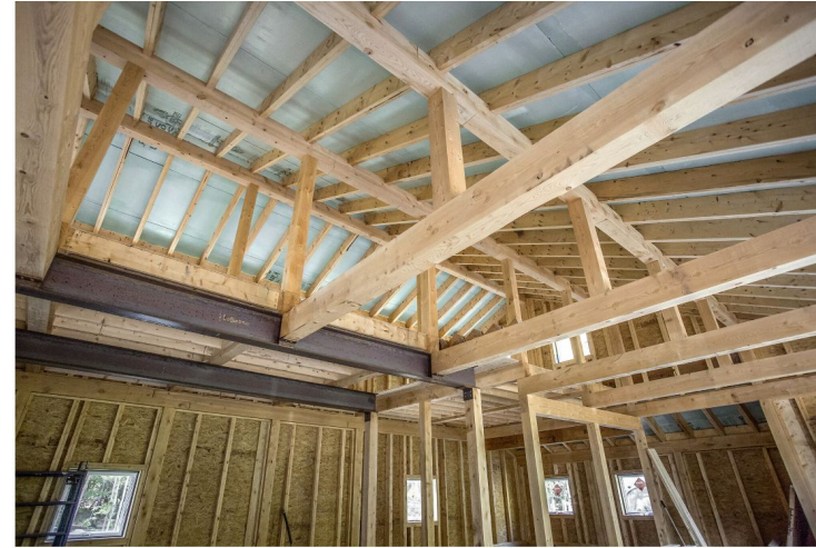
Interior of an efficient post and beam home, constructed by Burnham & Lobo Builders in Freeport. It was constructed using a continuous, air-tight, well-insulated exterior outer shell with R-35 walls and an R-65 roof. Photo by Tim Greenway.
